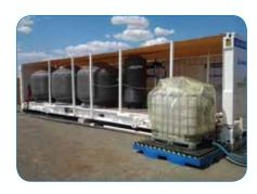
Waterco Micron fiberglass filters were installed conjunction with an ion exchange filter media to remove sodium out of the incoming water whilst adding calcium and magnesium. The end result is recycled water that is ideal for soil and plant health.
