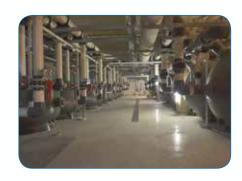
Glen Eira Sports and Aquatic Center (GESAC) features five separate pools, two water slides, and a fully equipped aquatic wellness area. The aquatic centre has been equipped with Waterco's Micron Air Scour Horizontal filtration system, which has resulted in a saving of between 25 and 35 percent of the backwash water.
