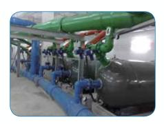
12 Micron MD6500 Commercial fiberglass filters and 11 Micron M5000 Commercial fiberglass filters purify over 4 million gallons of water at Asia's premier destination resort, Universal Studios on Sentosa Island in Singapore. The Micron M5000 filters are used for the water theme park (9,900m³ volume of water), while the Micron MD6500 filters are installed to service three different attractions,
