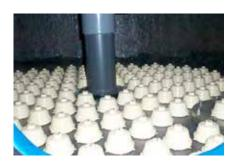
Nozzle Plate under drain system
